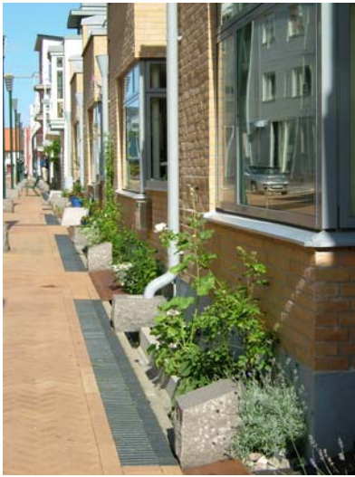
Downspouts draining into an open surface channel keep plants well watered (photo by Deb Guenther, Mithun)
