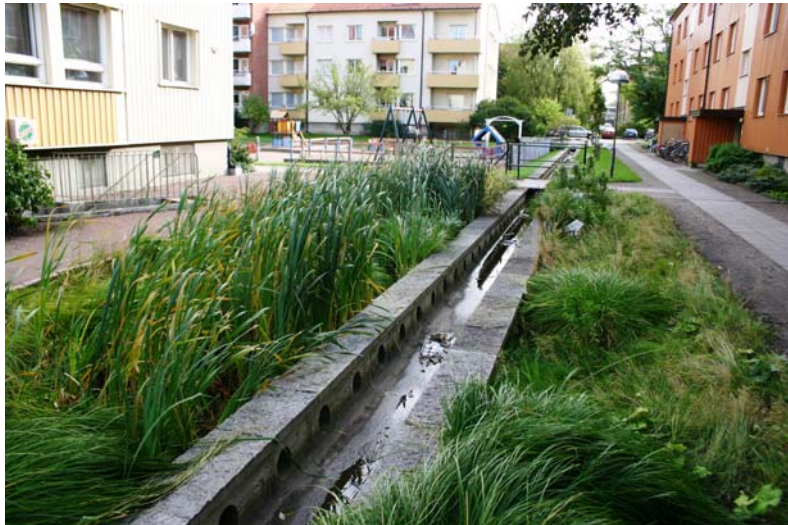
Channels in the Augustenbourg neighborhood of Malmö, Sweden are designed to drain water into surrounding wetlands during heavy storm flow (photo by Mark Brumbaugh, Brumbaugh & Associates)
